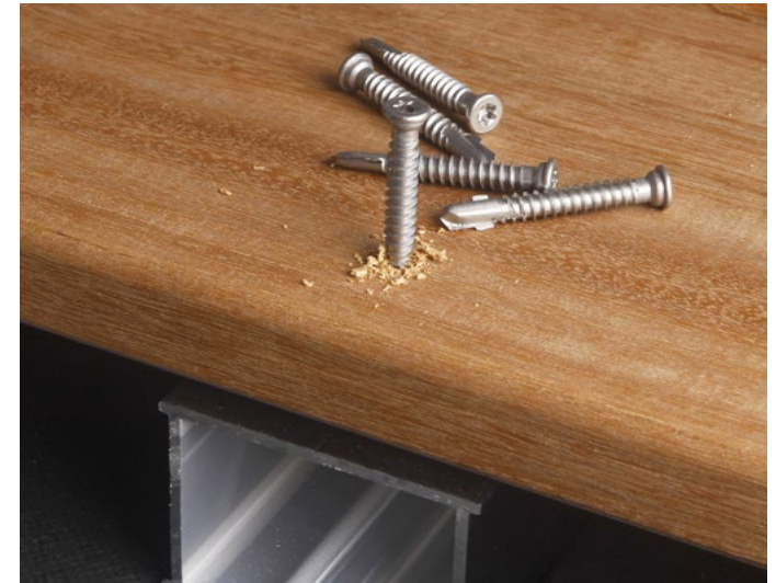
Fixing with Cobra inox screws
